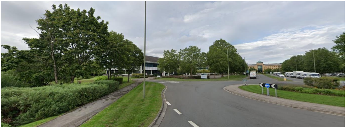
Existing buildings north of Riverside Way to be demolished.
